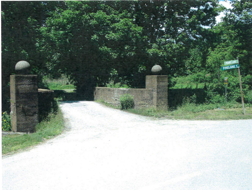
Roadway over the structure - Looking west
