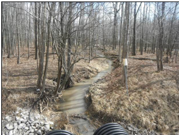
Photo 62: Reach 14-B, channel character, Miller Road cross culvert at point of discharge of roadside ditching system into the West Branch of Beaver Dam Drain.
