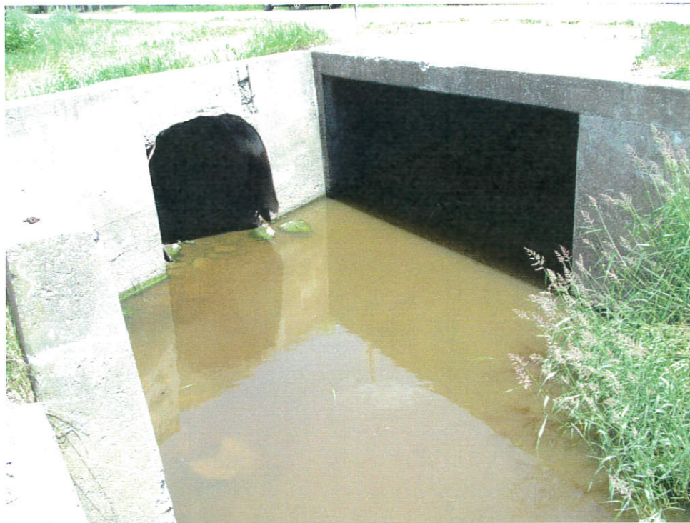
The west end of the structure
