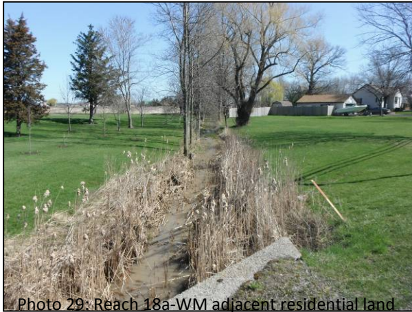
Photo 29: Reach 18a-WM adjacent residential land
