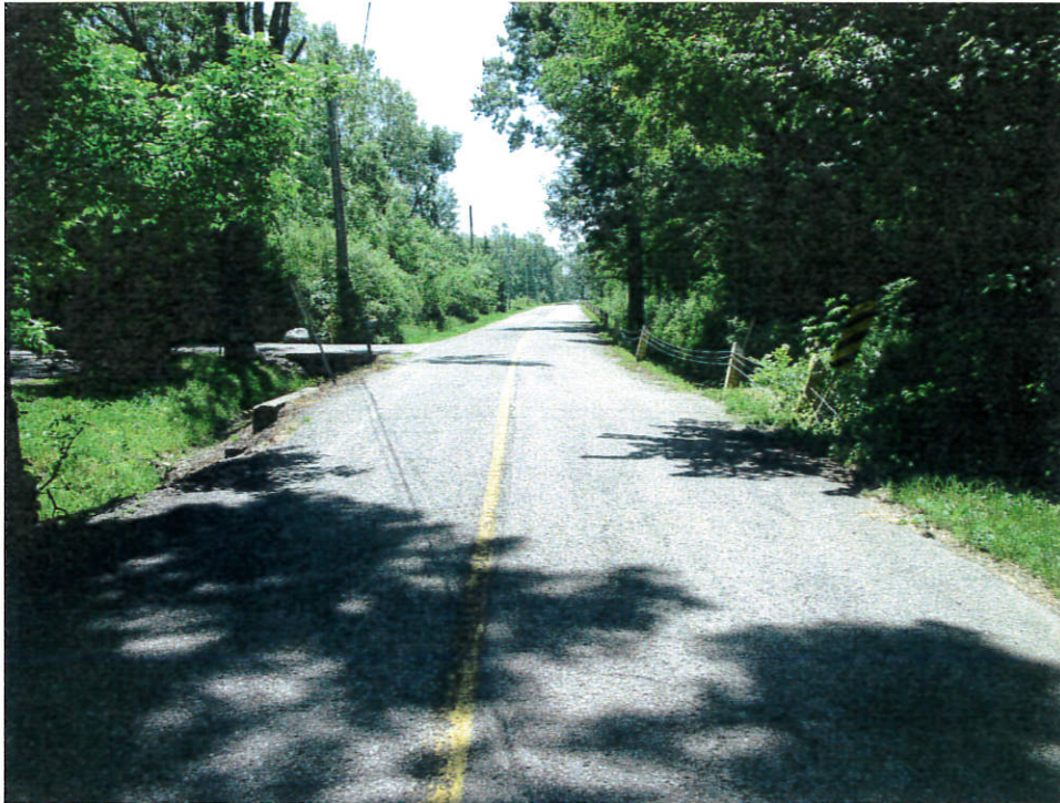
Roadway over the structure - Looking south
