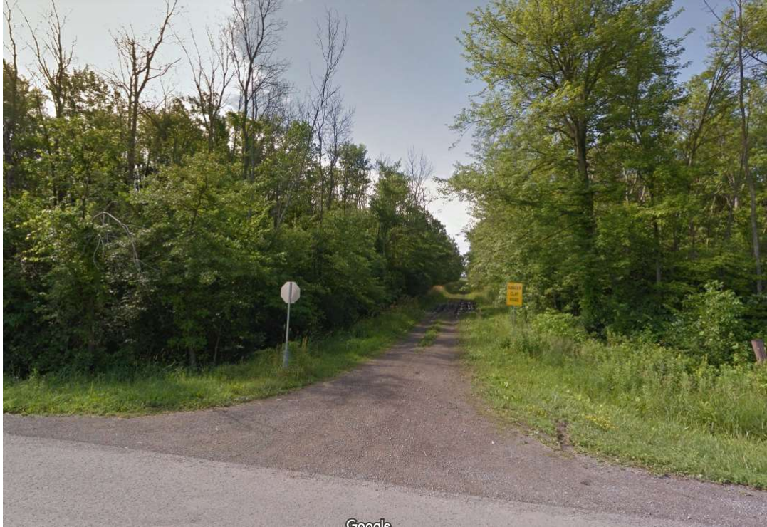
Figure 9 Wignell Drain Upper end @ Carl Road (clay) and Second Concession Rd.
