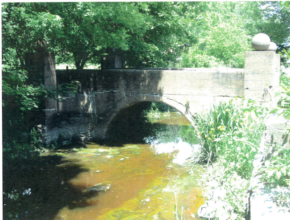
View of the structure, from the south side
