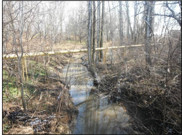
Photo 61: Reach 13-B, pipe crossing the drain and adjacent forest
