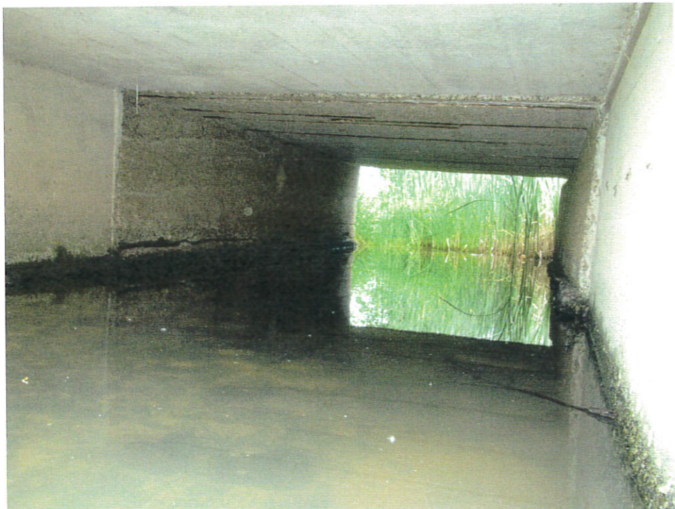
Viewing the interior of the structure from the west end
