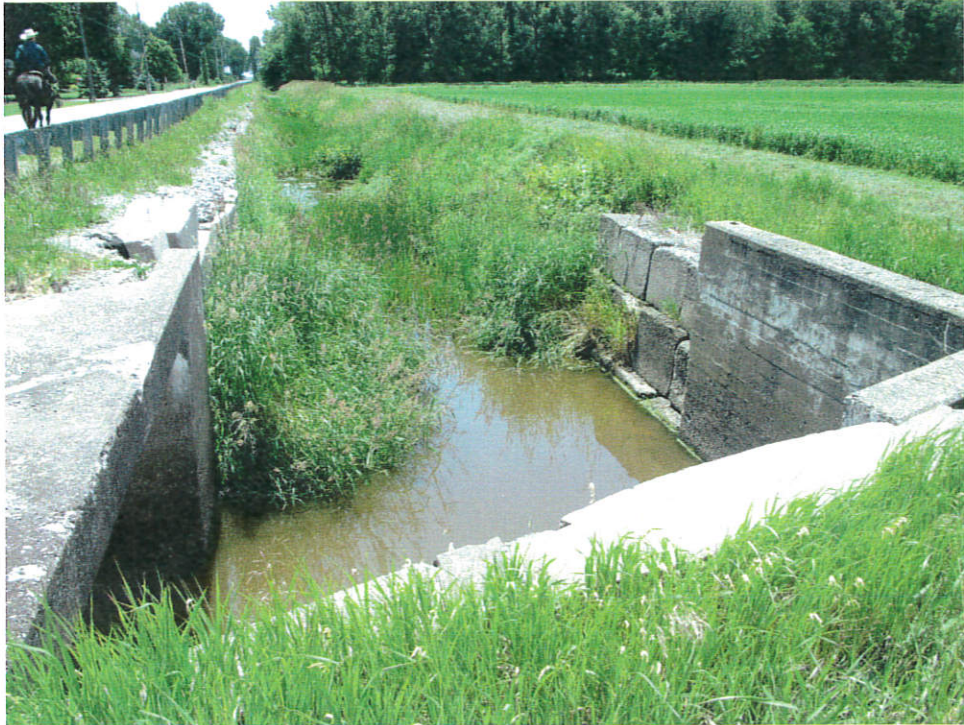
The west end of the structure
