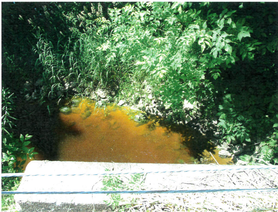
The west end of the structure
