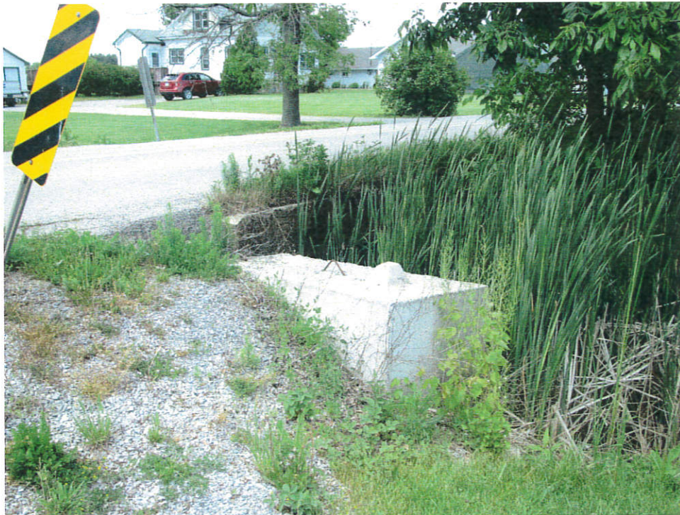
The east end of the structure
