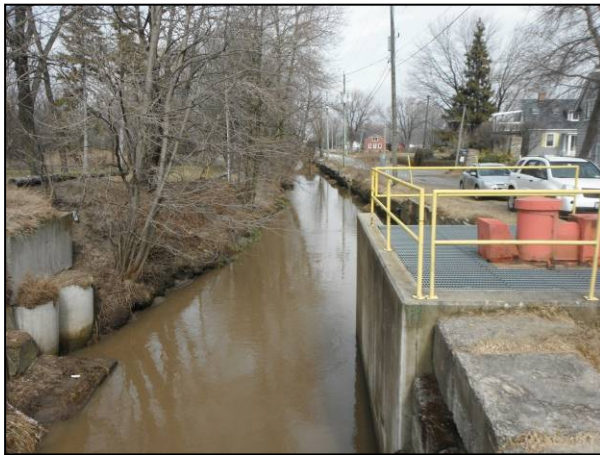
Photo 37: Reach 1-B, water control structure
