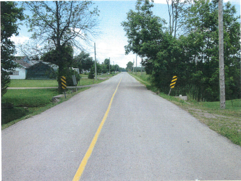
Roadway over the structure - Looking north
