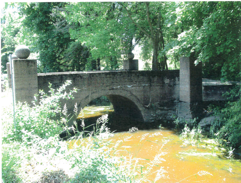
View of the structure, from the north side
