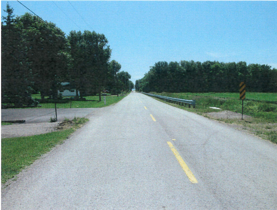
Roadway over the structure - Looking south
