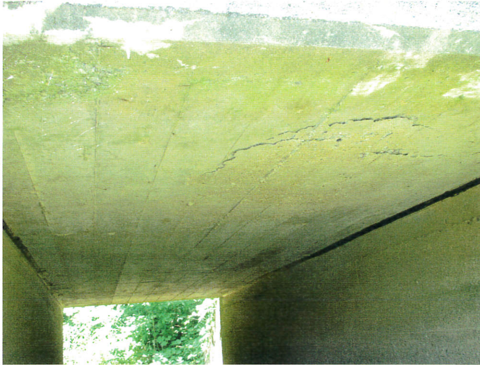
The underside of the structure
