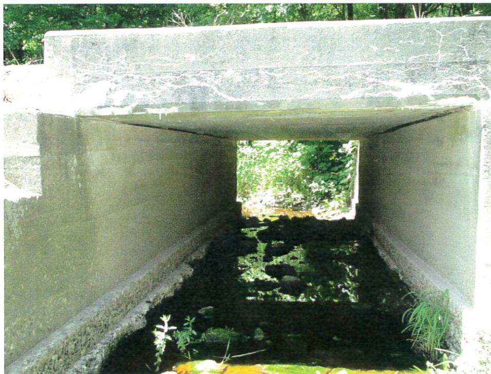
Viewing the interior of the structure from the east end
