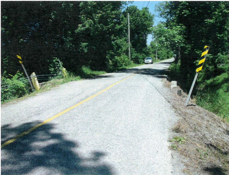
Roadway over the structure - Looking north
