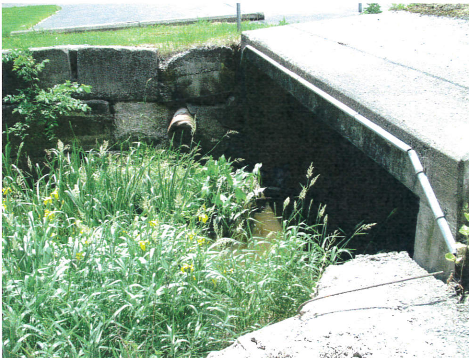
The east end of the structure
