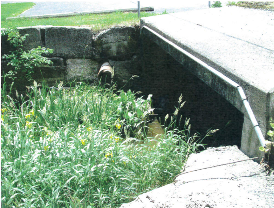
The east end of the structure
