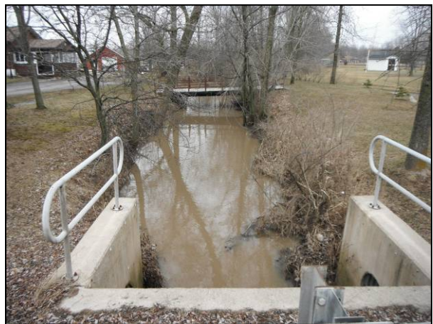
Photo 48: Reach 6a-B, Hwy # 3 culvert crossing headwall & lateral drainage (piped roadside ditching)pipinginterface. Former Geo. A. Schooley Award Drain. 16
