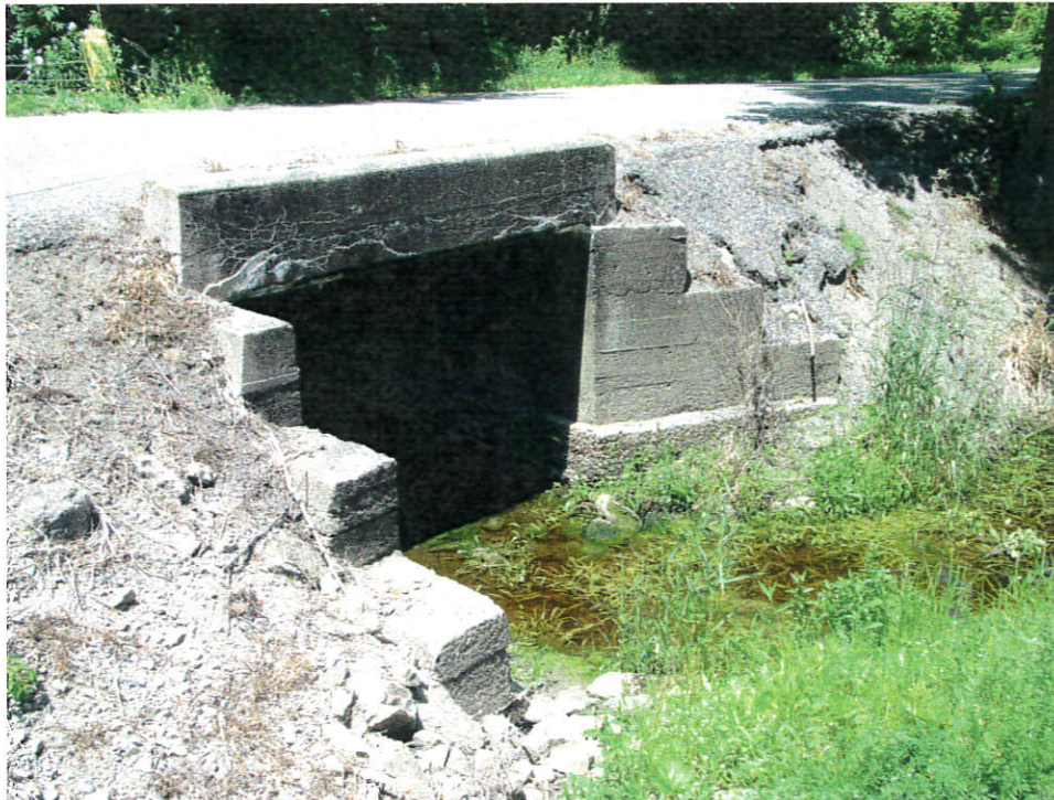
The east end of the structure
