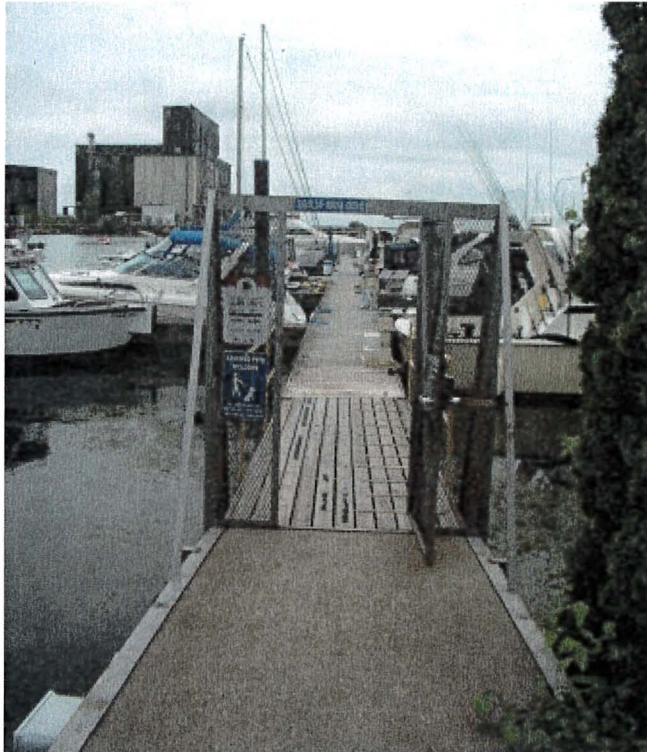
Photograph 17: Dock 2 – Access Gate. Front View
