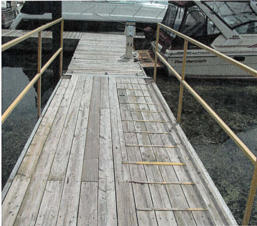
Photograph 3: Dock 1 – Access Gangway. General View.
