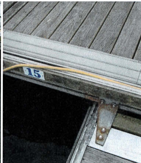
Photograph 110: West Main – Dock D. Base Plates Corroded in Finger 14/15
