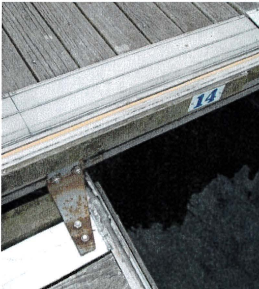
Photograph 110: West Main – Dock D. Base Plates Corroded in Finger 14/15
