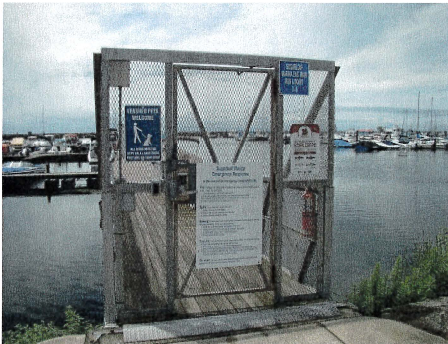
Photograph 30: East Main – Access Gate. Front View
