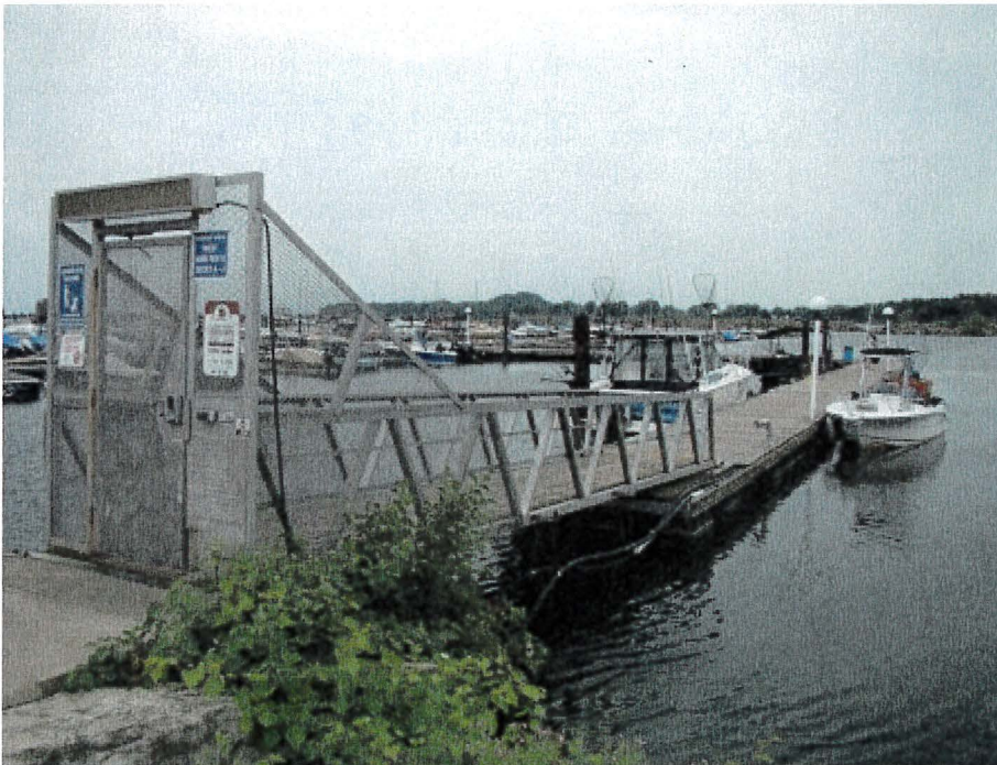
Photograph 68: West Main – Access Gangway. General View
