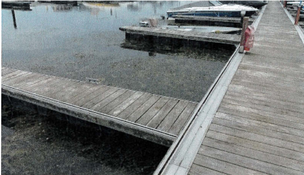
Photograph 155: West Main – Dock J. Very High Presence of Marine Vegetation in the Water
