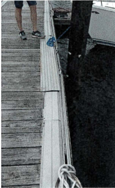
Photograph 127: West Main – Dock F. Pile 7. Steel Wire instead of Pile Guide. Dock Misaligned and Deformed
