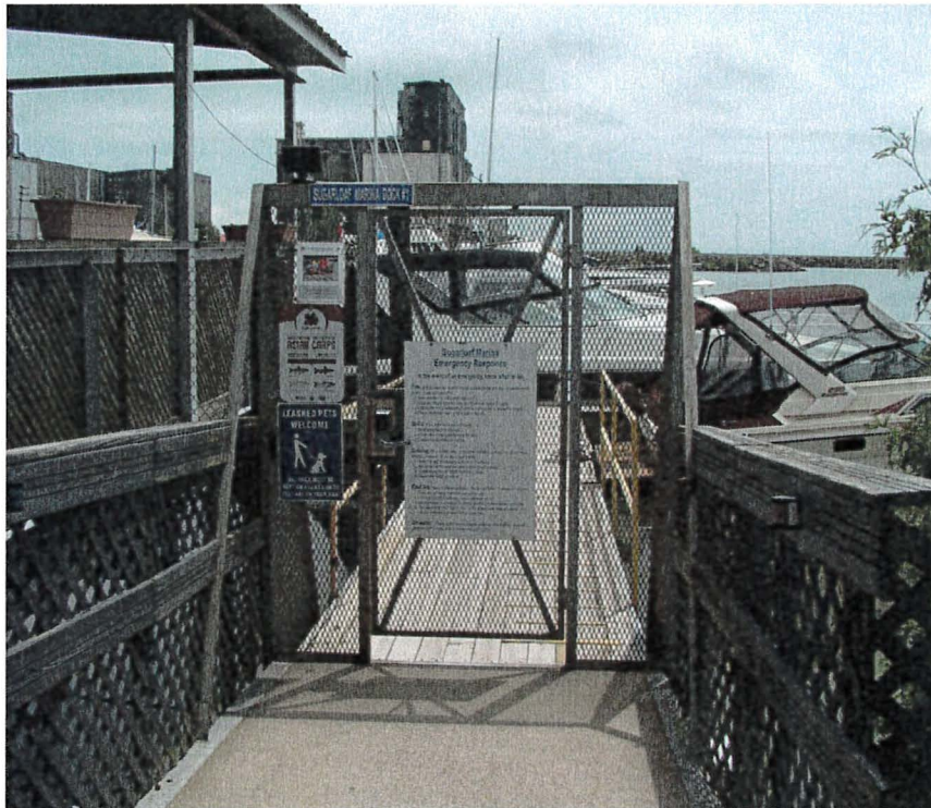
Photograph 1: Dock 1 – Access Gate. Front View
