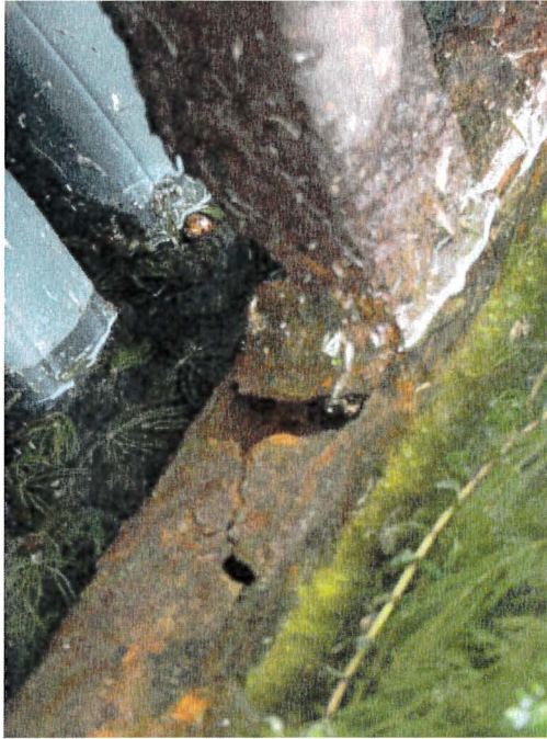
Photograph 55: East Main – Dock 4. Moderate to Heavy Corrosion of Steel Frame for Tubular Plastic Floats (3)
