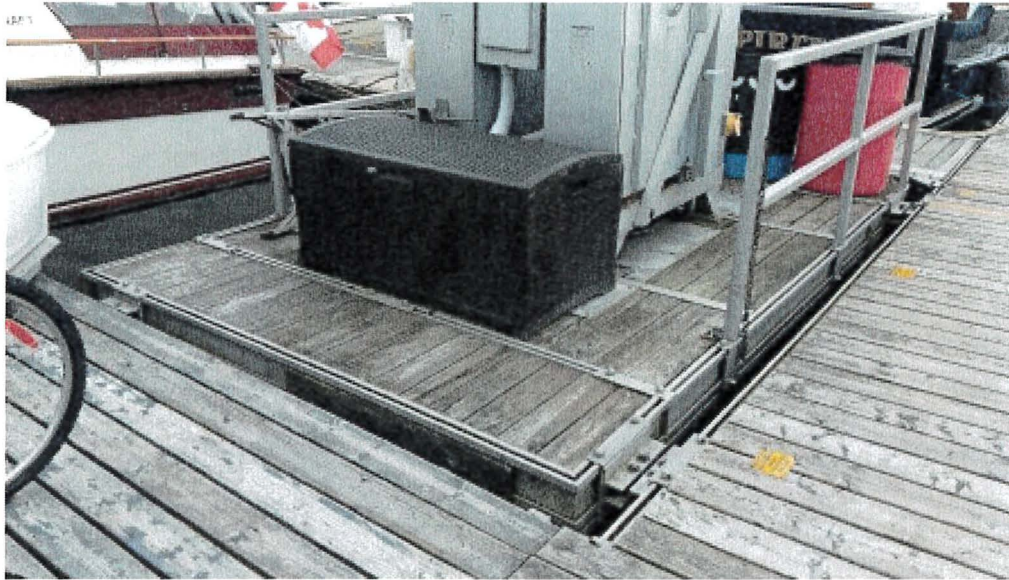
Photograph 79: West Main – Picnic Dock D-E. Different Settlement between Outer and Inner Sides
