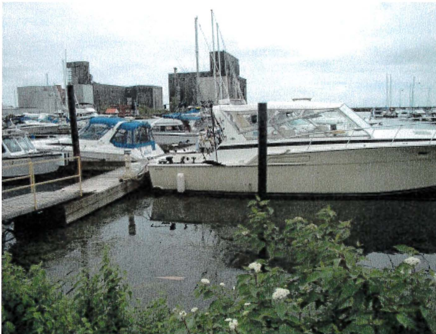
Photograph 44: East Main – Final Section. Different Float Types on Left and Right Sides. No Life Rings. No Fire Extinguishers
