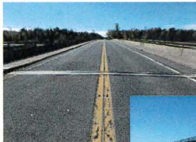
Townline Road Bridge – looking south
