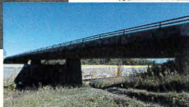
Townline Road Bridge – west elevation
